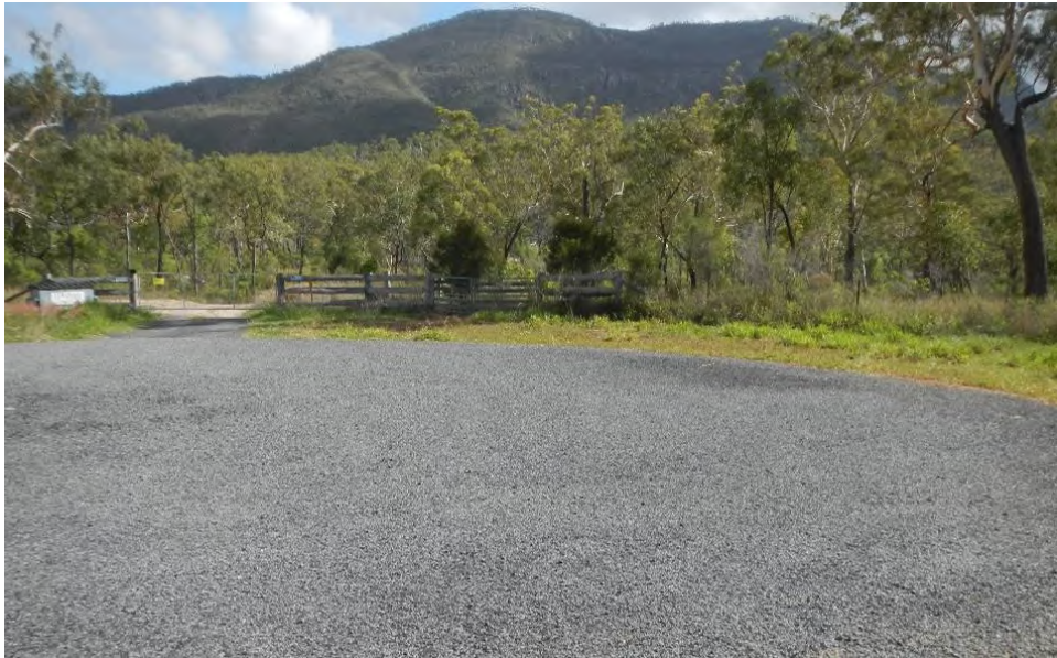
Figure 2. The entrance to the offset site through the gate and to the right of picture. The bitumen provides a useful barrier to weed growth, rendering the access to the property relatively easily managed in terms of weed control.
