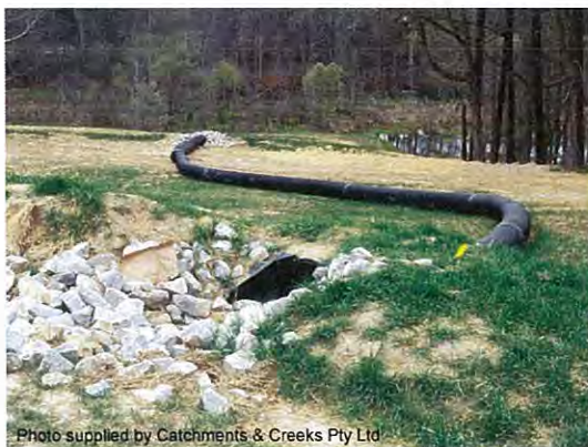
Photo 1 – Temporary Slope Drain with rock stabilisation at inlet and outlet
