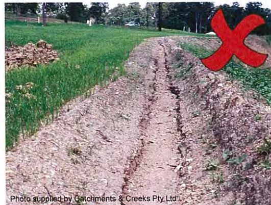
Photo 6 – Velocity-induced bed scour within a catch drain
