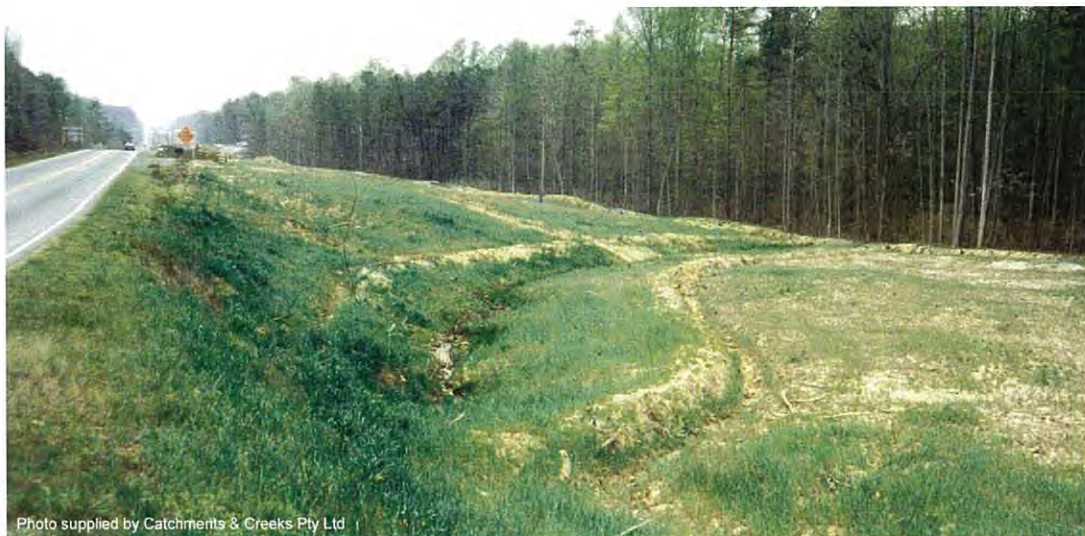
Photo 7 – Flow diversion banks placed each side of drainage line passing through road construction site
