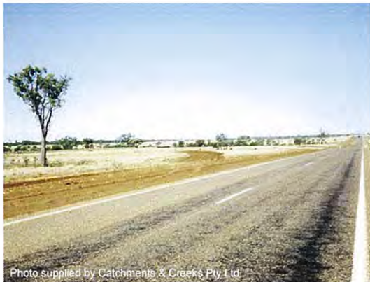
Photo 1 – Diversion drains (centre) collect stormwater from roadside table drains, then releases the water as sheet flow via a level spreader
