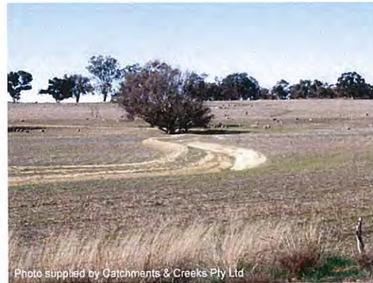
Photo 2 – Large rural catch drain (channel-bank)
