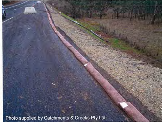
Photo 2 – Sandbag flow diversion berm used to minimise surface flow over a recently seeded embankment
