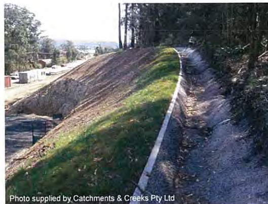
Photo 4 – Permanent catch drain
