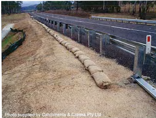
Photo 1 – Flow diversion berm used to minimise road runoff flowing down a steep, unstable section of the embankment
