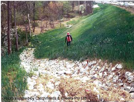
Photo 3 – Rock lined catch drain
