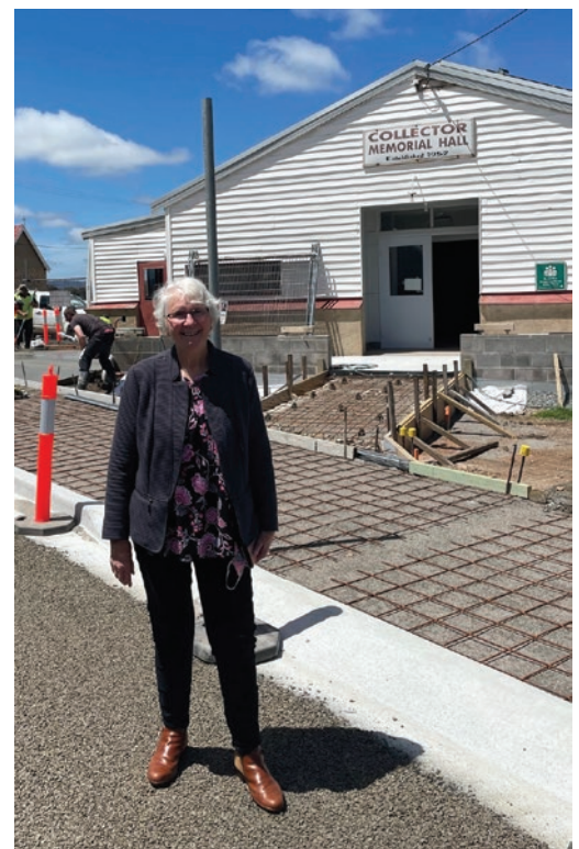
Collector Community Hall improvements
