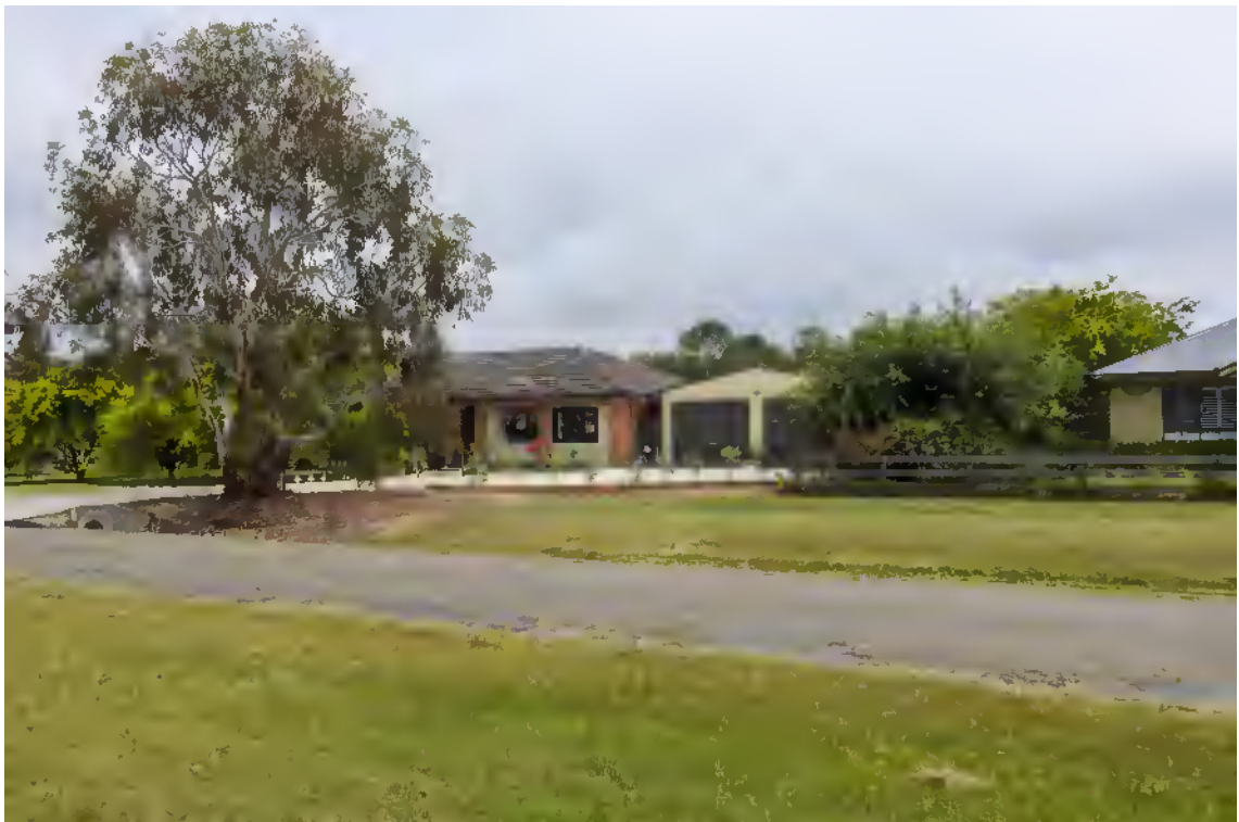
Figure 87 Test Site - Location R
