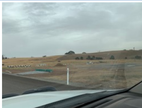
Photo 12: Example of sediment and erosion controls installed along Lerida Road South.
