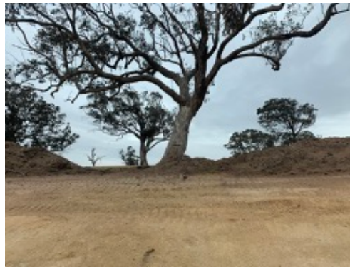
Photo 8: Topsoil stored for rehabilitation.
