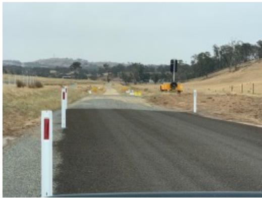
Photo 13: End of project upgrade works along Lerida Road South.
