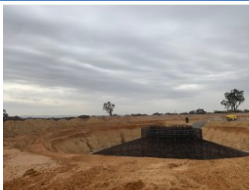
Photo 4: Wind turbine fountain works under construction.
