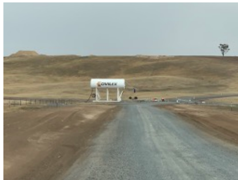
Photo 10: Dedicated water cart filling tank.
