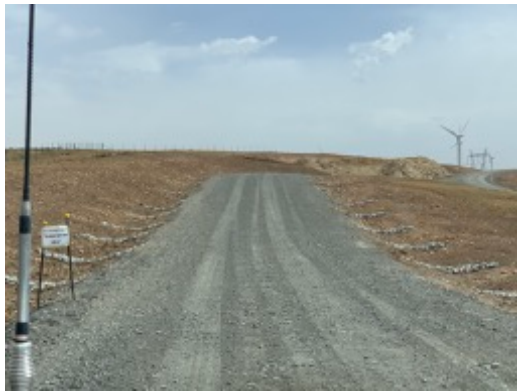
Photo 25: Example of completed site access road towards substation.
