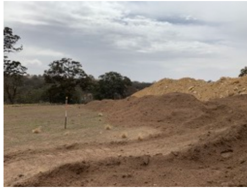
Photo 20: Top soil retained in wind row for rehabilitation purposes.
