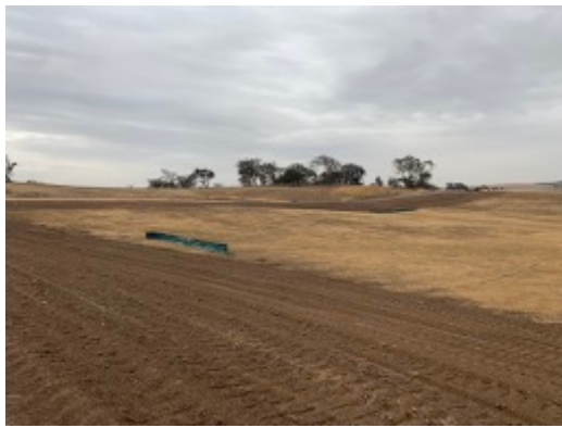
Photo 9: Rehabilitation of internal access tracks is limited to final dressing of topsoil and contouring. Sediment controls remain in key drainage points. Seeding has not been undertaken due to prolonged drought conditions on site.
