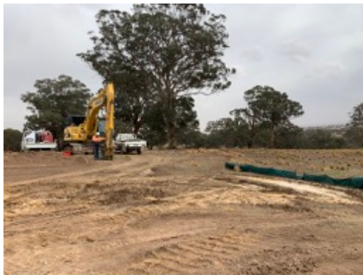
Photo 21: Sediment fencing progressively installed into new work areas.
