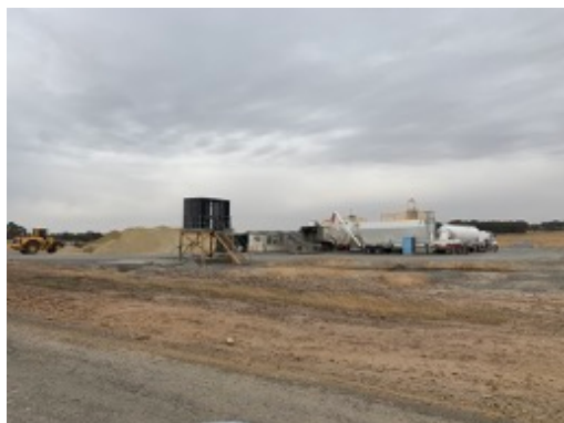
Photo 1: Concrete batch plant with sedimentation basin in centre foreground.
