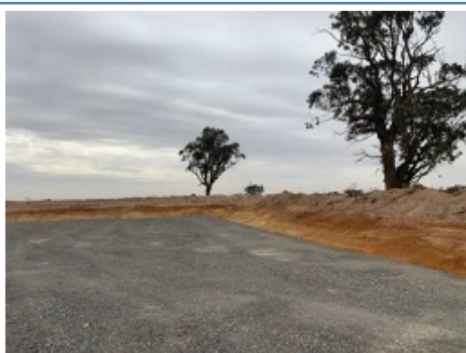
Photo 5: Evidence of wind turbine hardstand area, including v-drain and stockpiled topsoil.
