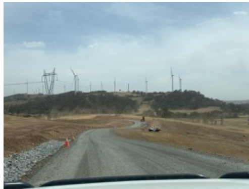
Photo 26: Example of completed site access road and rock lined v-drain.
