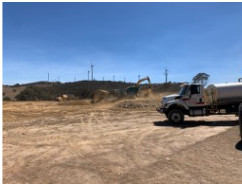
Photo 32: TransGrid substation crushing operations and water cart.
