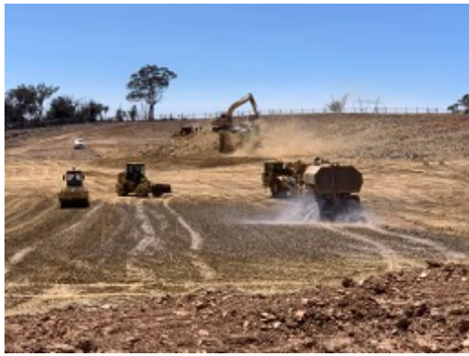
Photo 37: TransGrid substation works. Dust from crushing plant settling on site.
