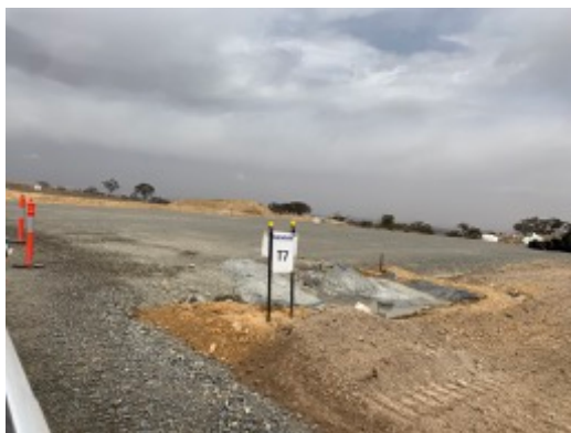
Photo 23: General site photo of WTG 17 hardstand. .
