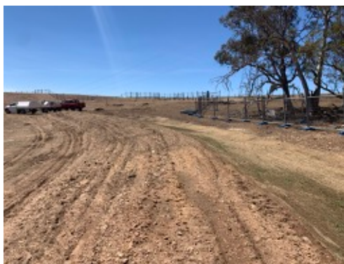
Photo 34: Upslope clean water diversion drain above TransGrid substation.
