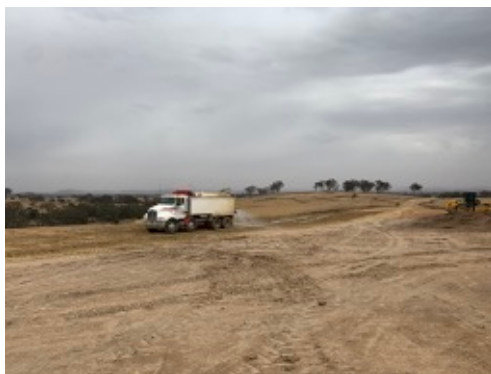
Photo 18: Water cart in operation for dust suppression.
