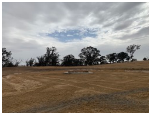
Photo 2: Example of wind turbine foundation preparation works.
