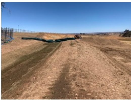
Photo 33: Upslope clean water diversion drain above TransGrid substation.
