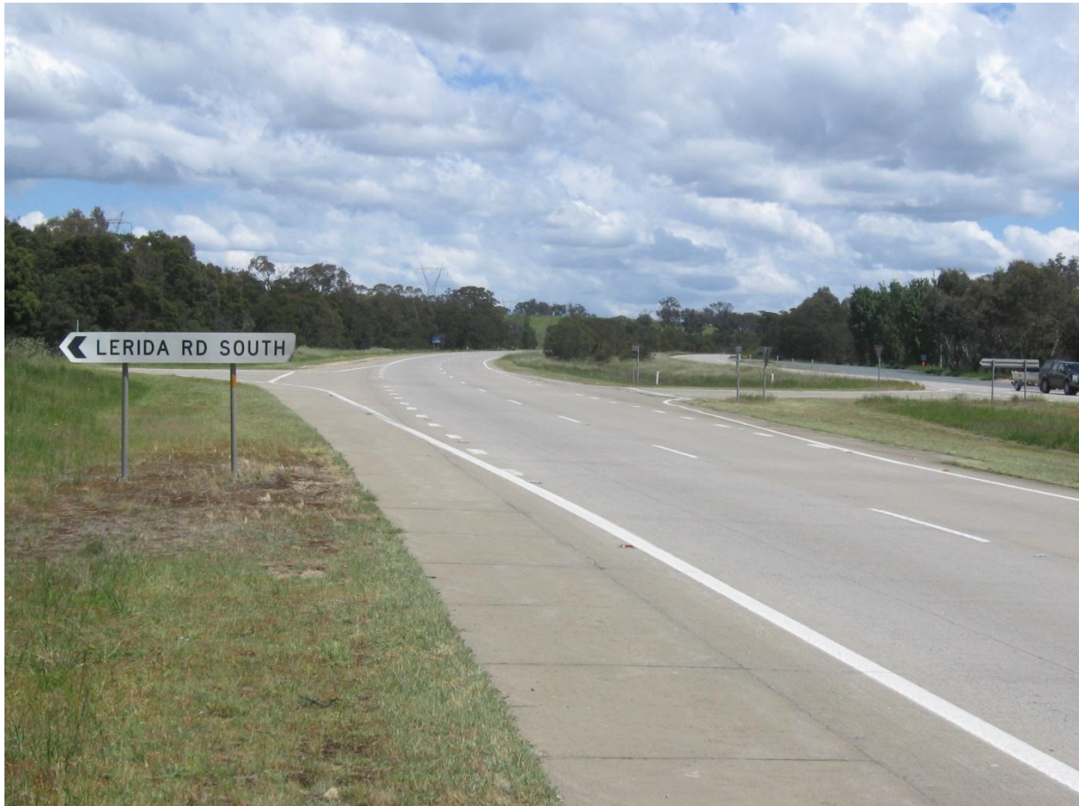
Figure 4 Site Access – Hume Highway / Lerida Road South intersection
