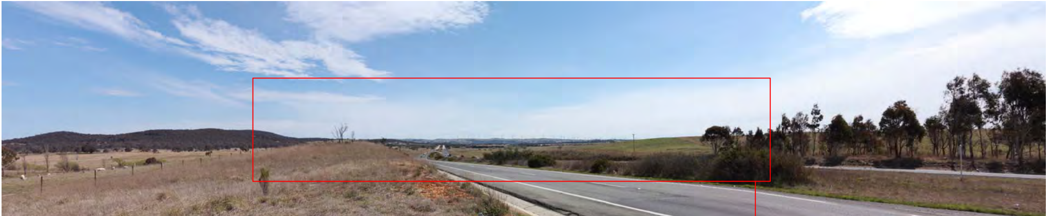
Photomontage Viewpoint 05 Federal Highway North of Collector, view west toward proposed Collector Wind Farm
