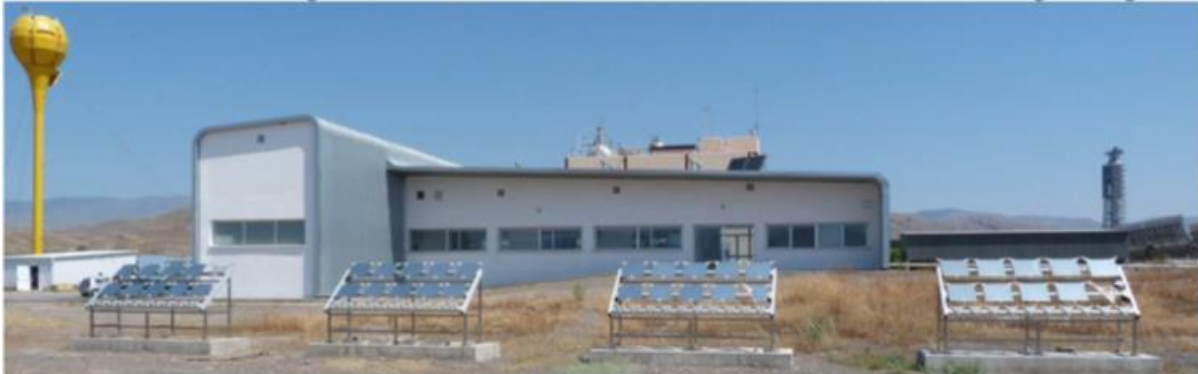
Figure 6. Structures 1 to 4 (from left to right) at OPAC's outdoor exposing area (25)
