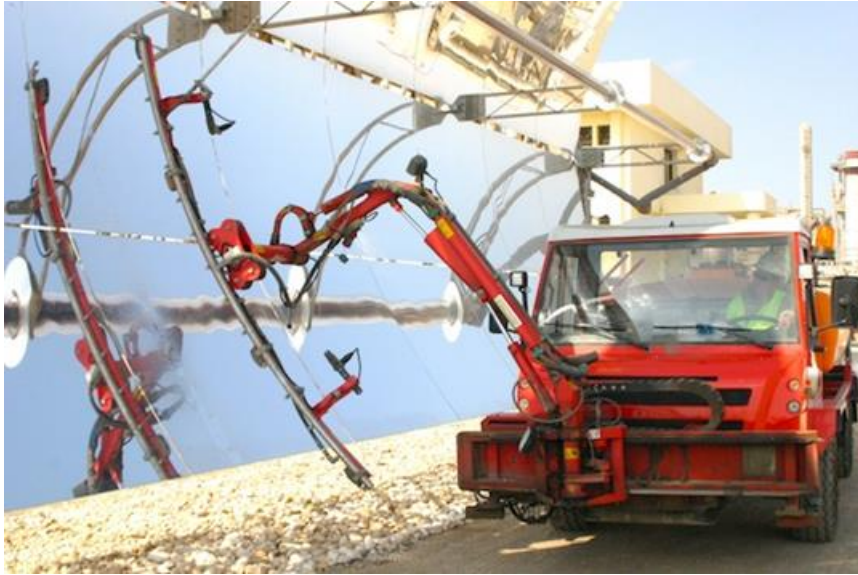
Figure 17. Water washing system used in Kuraymat Solar Power plant (33)
